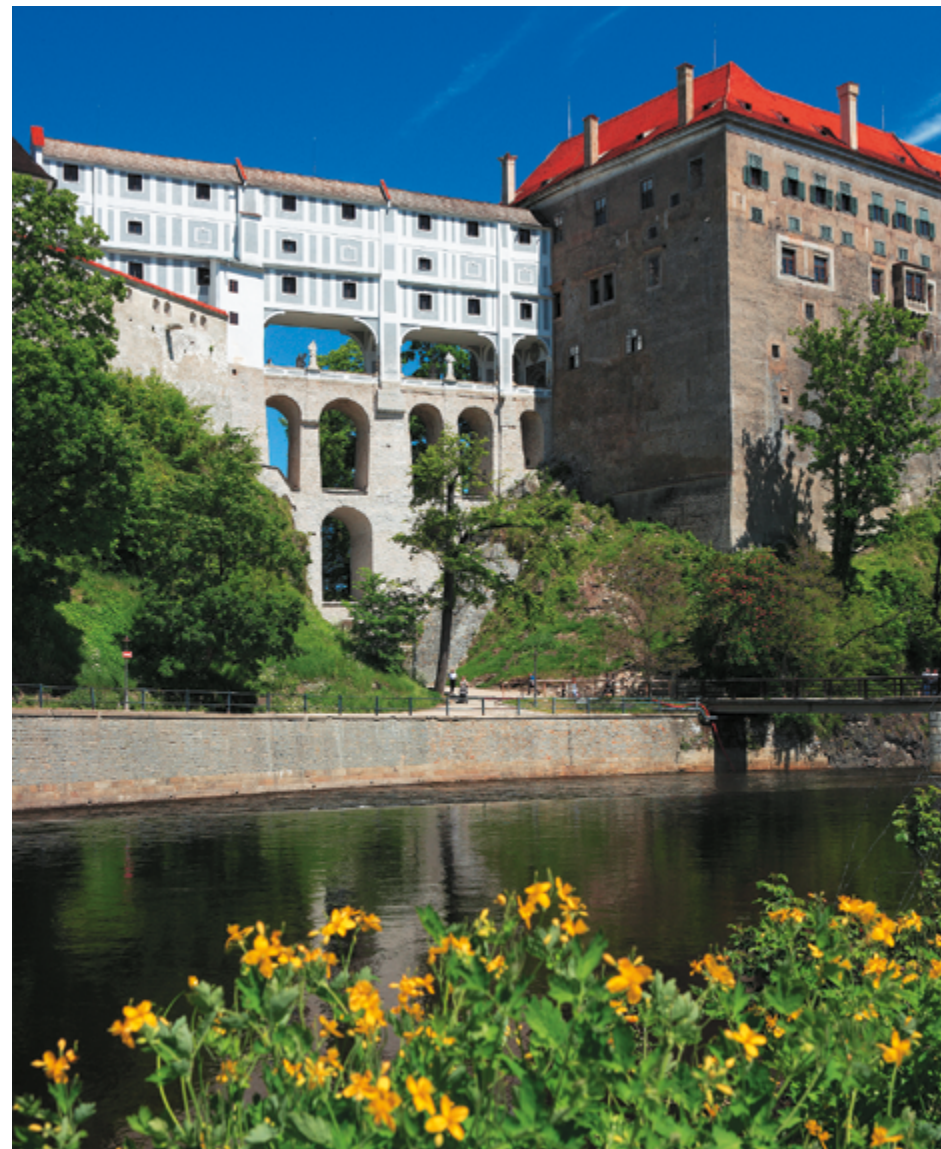
The Cloak Bridge connects the fourth and the fifth courtyard. In addition, it supports sheltered corridors that are directed to the Baroque Theater and Castle Gardens.
